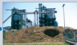
Centrali termiche a biomassa Biomass power stations
